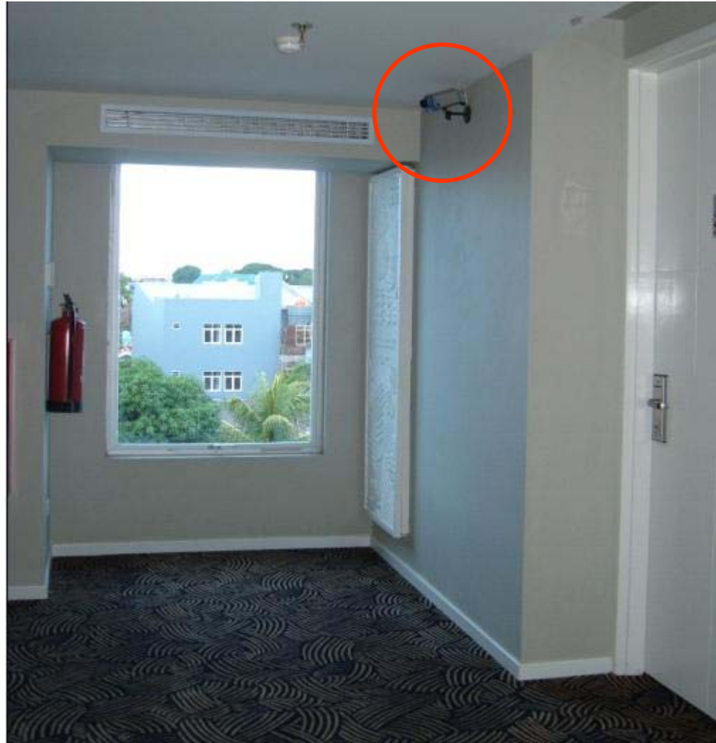
IP camera at corridor
